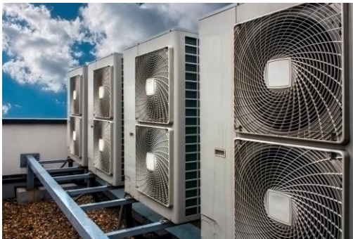
Figure 1: filter unit for an air conditioning system.
